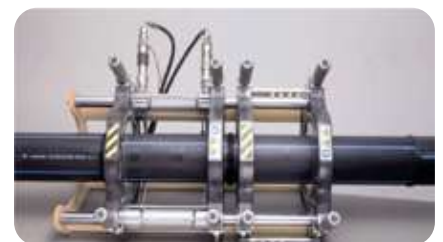
Stage 5: welding with element in pressure.
